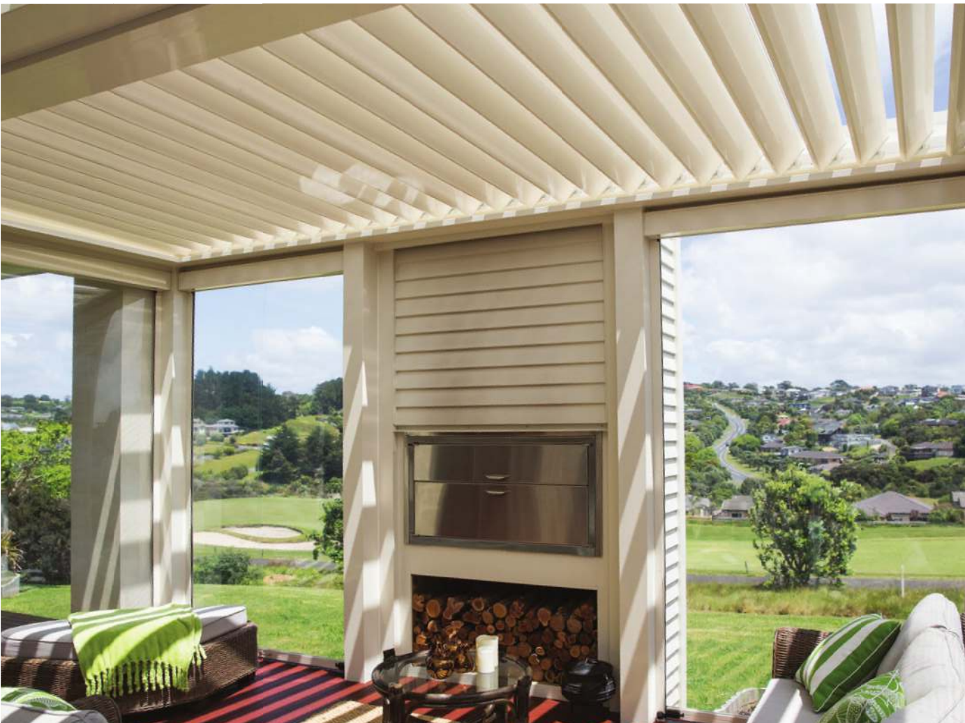
OPENING ROOF WITH CLEAR PVC BLINDS
